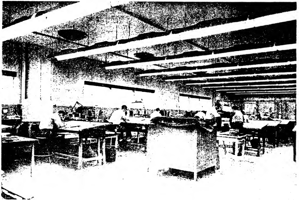
Increased demands on the Tool & Die plant's engineering services by Sheaffer's growing list of customers has made it necessary to enlarge the engineering department. The department has taken over the area formerly occupied by the welding department which was moved to an adjoining building.
